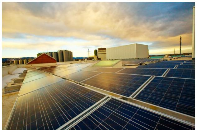
Photo: New Belgium Brewing **More Beer, Fewer Watts:** Solar panels at the <u>New Belgium</u> <u>Brewing Co.</u> in Fort Collins, Colo., supply 3 percent of the plant's electricity. The brewery is participating in the city's long-term plans to create a net-zero-energy downtown district and to become carbon neutral by midcentury.
