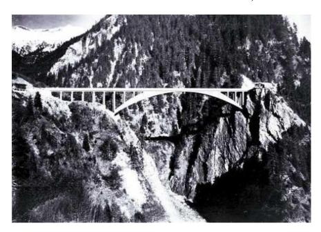
The bridge is a three-hinged arch with a span of d=90 meters and a rise of h=13 meters. The total weight of the bridge is estimated at W=7500kN.
