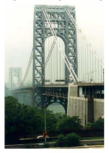
The cables carry the weight of the suspenders, deck and traffic, which may be calculated as follows:
