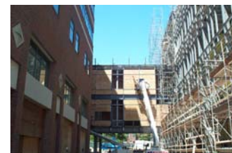
New Life Sciences Building under construction
