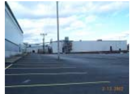
View from rear parking - High Bay on left, Storage straight ahead
