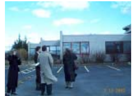
View from front parking to Office
