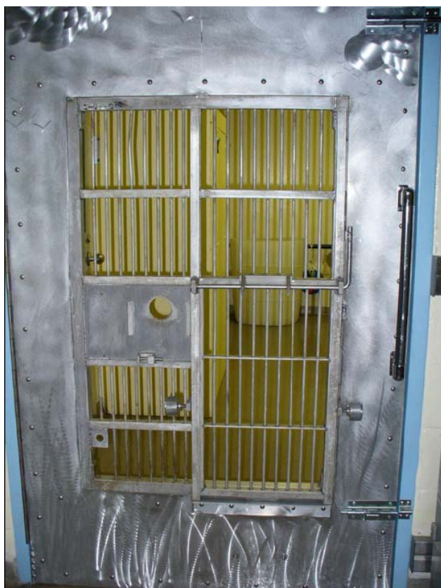
Figure 1: The door constructed to safely transfer baboons in and out of the enrichment room.
