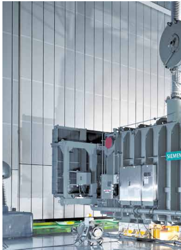
Converter transformer for the Three Gorges HVDC project 284 MVA, 1-ph/2-w unit
