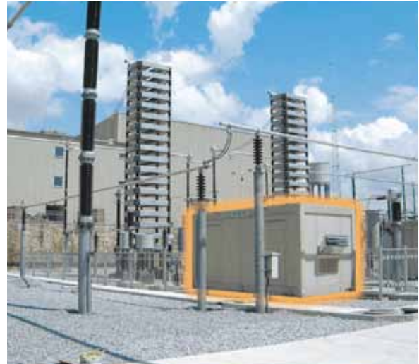
Fig. 5.4.3-1: Active DC filter on site (Tian Guang HVDC project)
