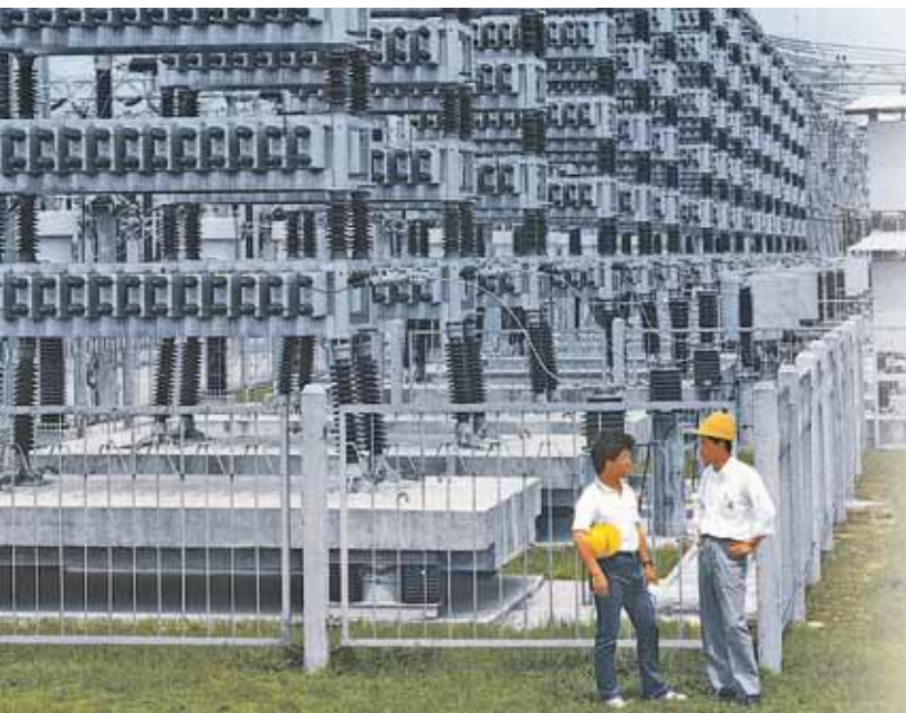
Fig. 5.4.1-2: AC filters and capacitor banks of Gezhouba/Shanghai
