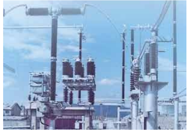
MRTB at Tian Guang/China DC switchyard
