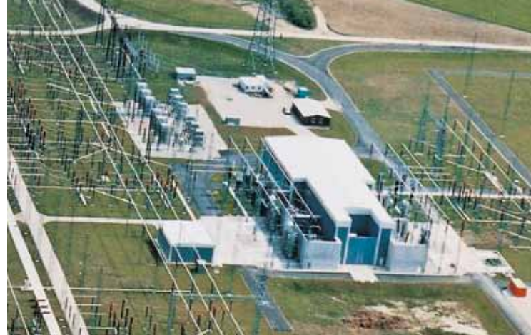
Fig. 2-3: Back-to-back converter Station Vienna Southeast
