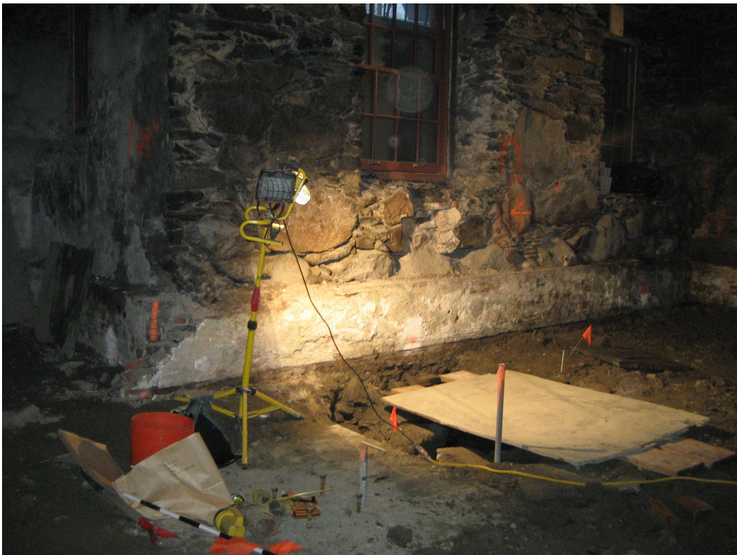
Figure 6. View of the three textures of the foundation wall: flat stones, brick, and stone rubble.
