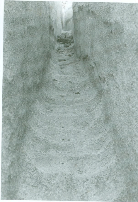
Fig. 10. Marks of dolerite hammers in one of the lateral trenches next to the Unfinished Obelisk at Aswan.
