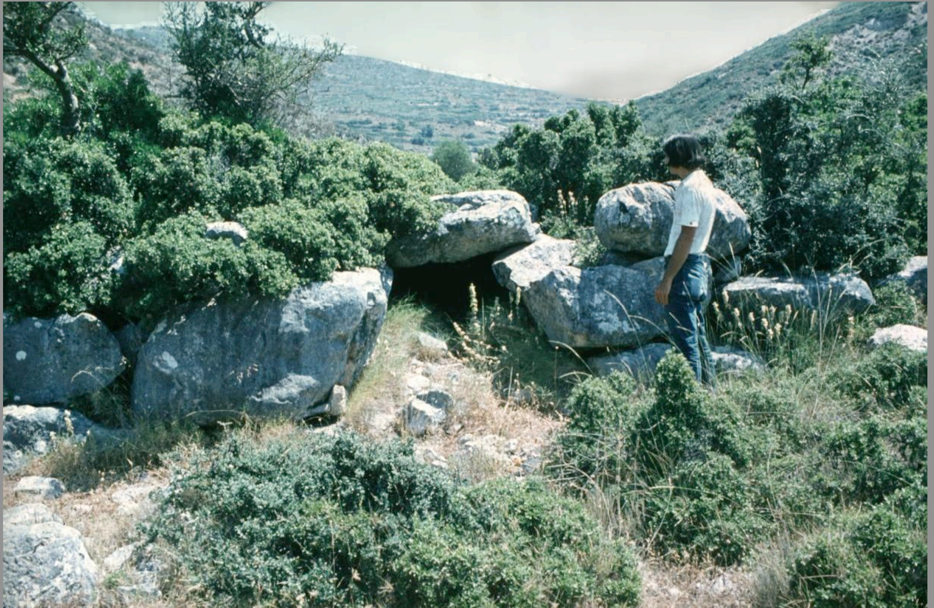
corbel-vaulted culvert running under roadbed
