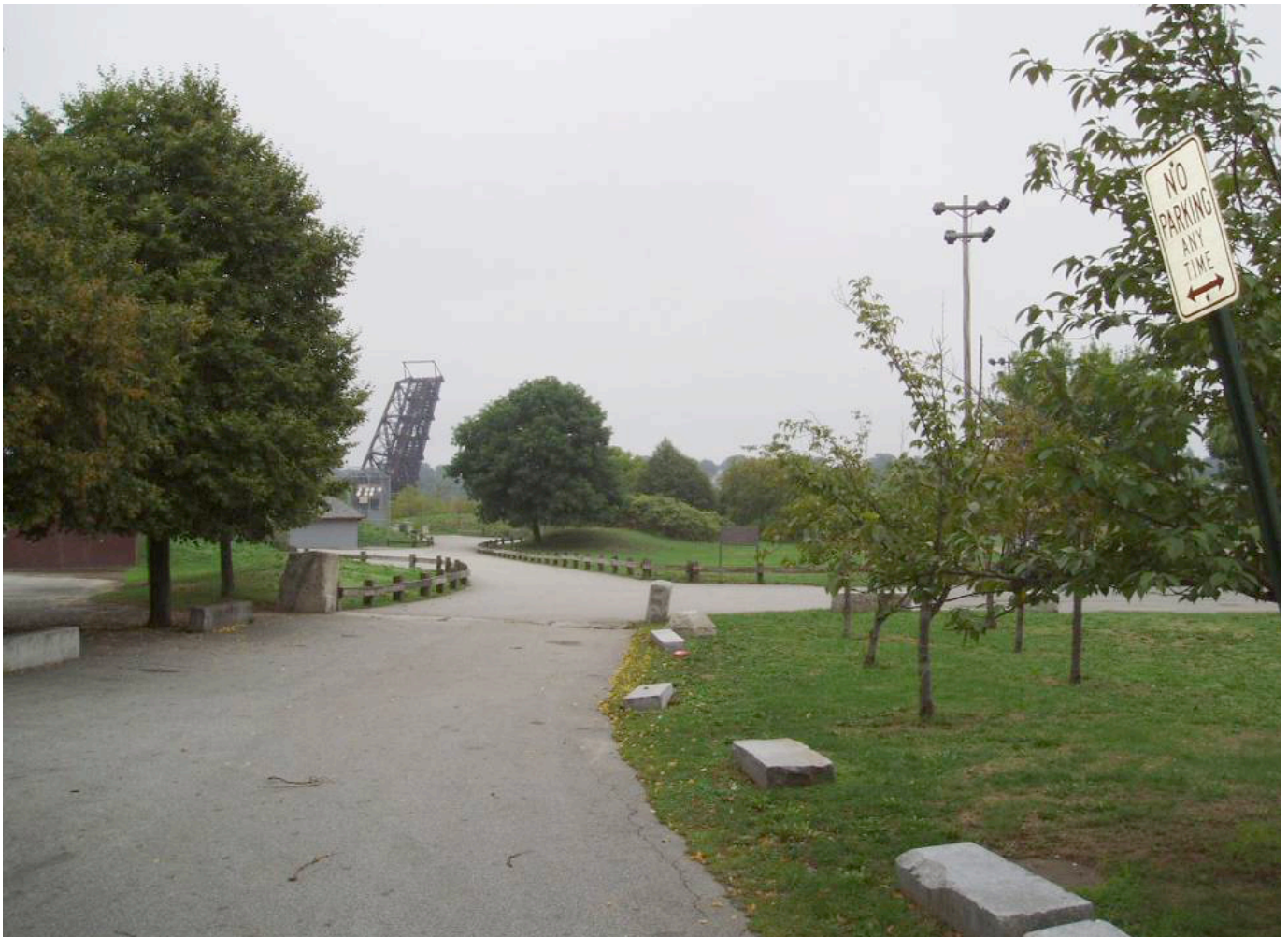
Crook Point Facing Schertzer Rolling Lift Bridge From Entrance
