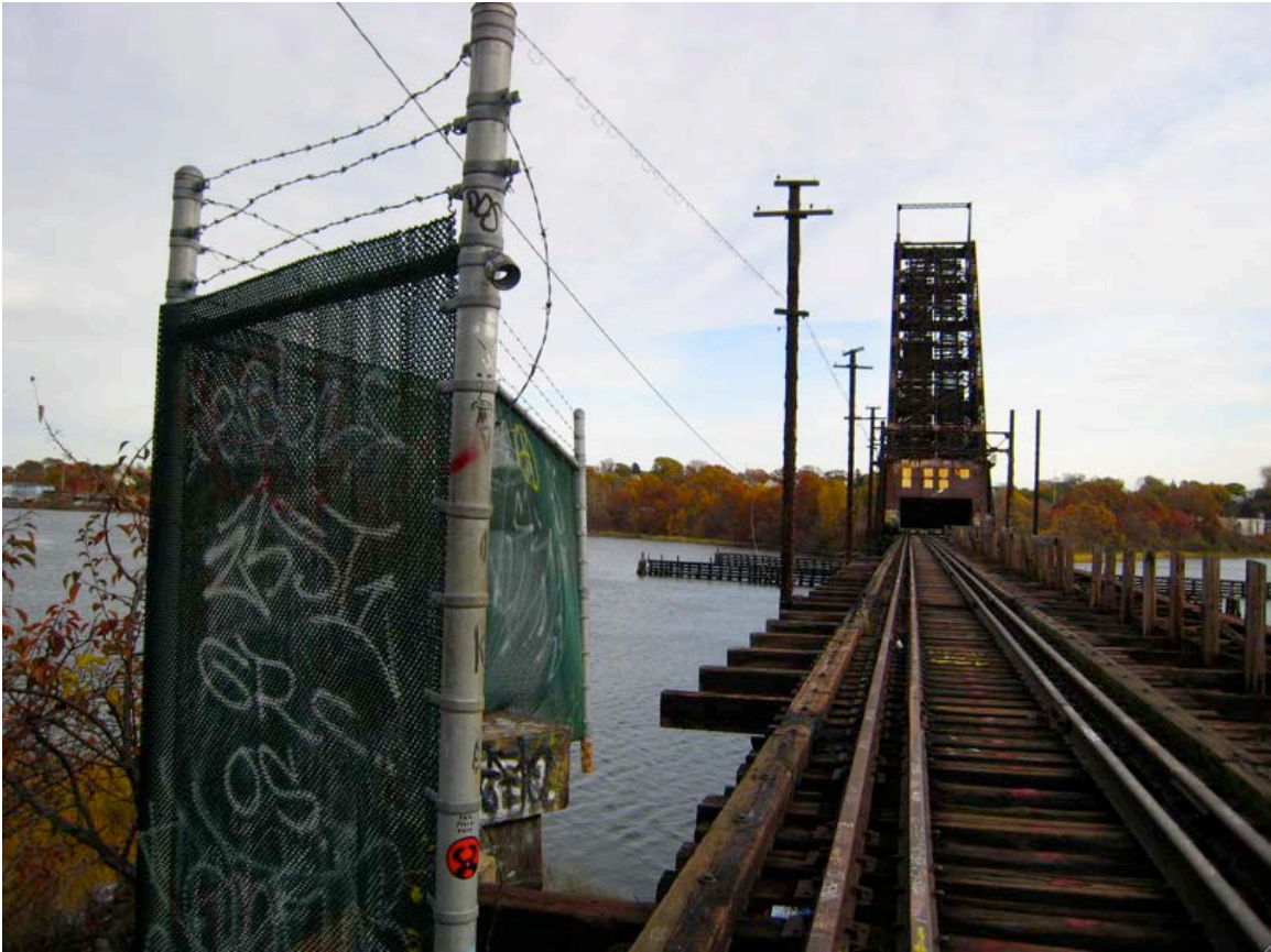
Barbed-wire fence almost surrounding bridge.
