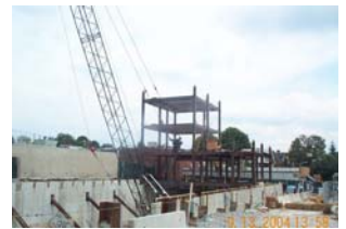
New Life Sciences Building. Steel construction began in September.
