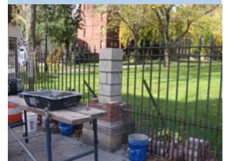
Rebuilding brick piers on the Main Green
