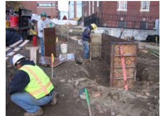
Forming concrete benches at the south end of The Walk
