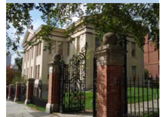
Fence and gate restoration at the Main Green
