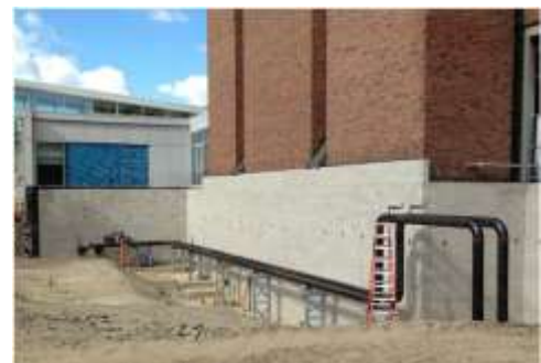
Utility of relocation & fire rated wall installation
