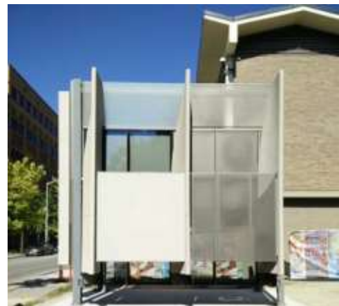
Mock up of exterior materials
