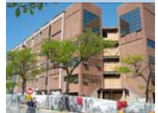
The J. Walter Wilson renovations are underway.
