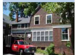
Work on the Brown-to-Brown houses has commenced.
