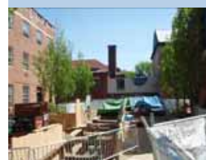
Utility work between Faunce House and Hunter Lab.
