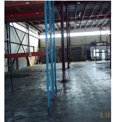
Under Construction Library Storage area 10 Park Lane.
