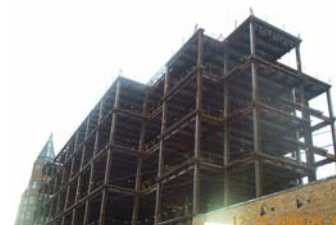
New Life Sciences Building under construction.
