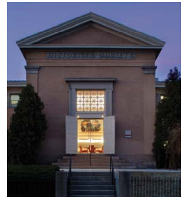
Cabinet Building—Renovated offices for Population Studies and Training Center opened this past Fall.
