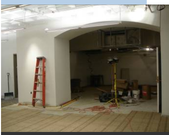
Renovation of the Brown Bookstore
