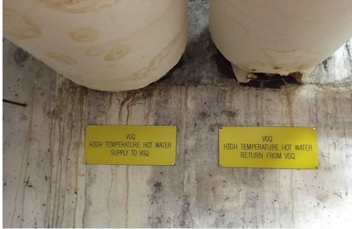
Example Wall Piping Penetration Tag
